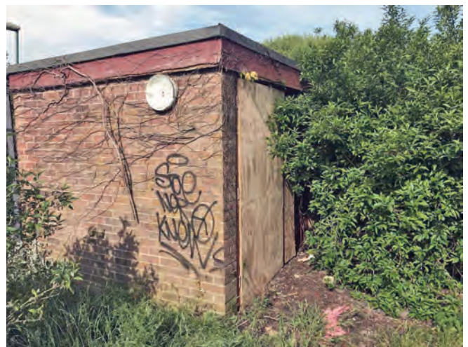
The emergency exit
